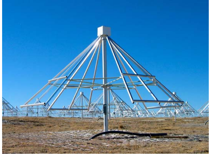
Figure 6: Antenna stand in field.
